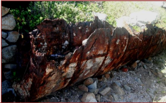
Photo 95. Boiler remains at the Copper Mine.
