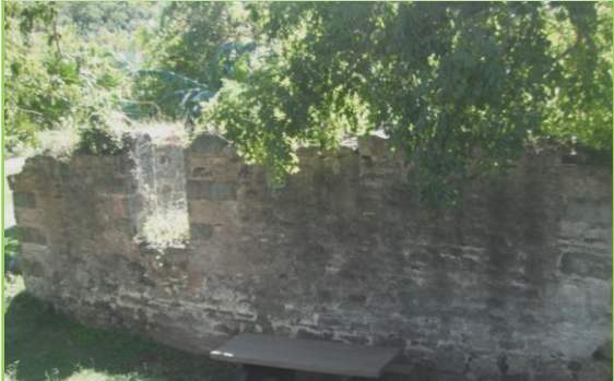
Photo 77. Nail Bay I Sugar Works.
