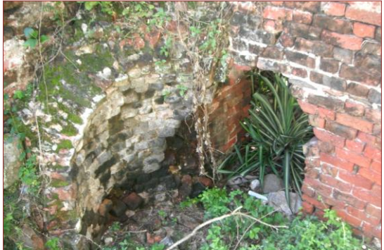
Photo 78. Nail Bay I Sugar Works.
