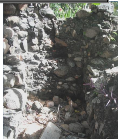
Photo 85. Nail Bay II Sugar Works.
