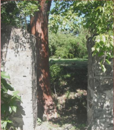
Photo 75. Nail Bay I Sugar Works.
