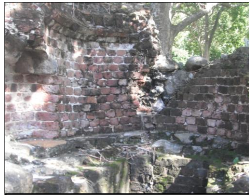
Photo 84. Nail Bay II Sugar Works.
