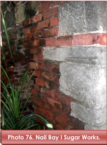
Photo 76. Nail Bay I Sugar Works.
