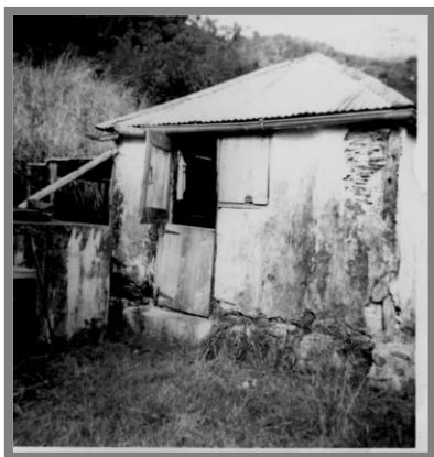
Photo 37. Example of wattle and daub house on JVD. In the top right hand corner of the house, the exposed wattle is visible.
